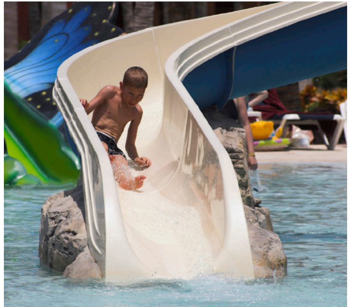
This slide exit is almost too vertical. A participant coming down head first could hit the concrete bottom.
